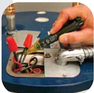
Because circuit breakers can be mismarked, always check the incoming power wires with a voltmeter or circuit tester to make sure the circuit you are working on is OFF.
