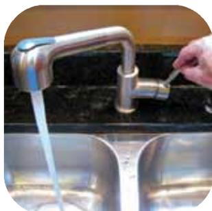
Open a nearby hot water faucet. At first, you'll just get air from the faucet, then sputtering, and finally, a full flow. Then, let the "hot" water run full for three minutes to ensure the tank is completely full. The tank must be completely full of water before connecting electric power or you will burn out (dry fire) the upper heating element.
