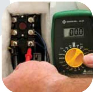
If you have some hot water, but not as much as you're used to, use a voltmeter and check the incoming voltage. See the wiring diagram and the water heater's label for power (voltage) requirements. Also, check the temperature setting on both thermostats—see Step 6.
