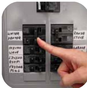
Locate the circuit breaker marked "water heater" and turn it OFF. Some homes use fuses which should be removed. Your water heater may also have a disconnect switch which should also be turned OFF.
