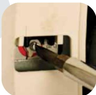
The upper and lower thermostats are both set at the recommended temperature setting of 120° Fahrenheit at the factory. Higher temperatures increase the risk of scalding. See the Installation Instructions and the water heater's labels for detailed instructions and important safety information about scalding.
