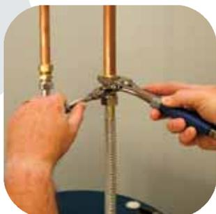
Install the hot and cold water lines. The water heater's inlet and outlet connections contain non-metallic parts. Don't solder pipe directly to these connections. Instead, solder threaded adapters to short pieces of pipe so that soldering is done a foot or so from the water heater connections. Open the cold water supply valve and fill the tank.
