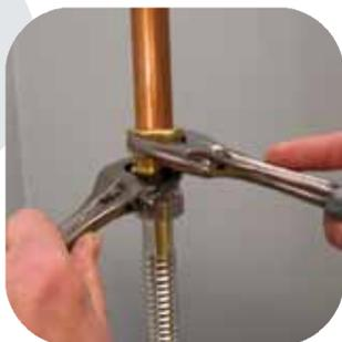
Check the water connections for leaks. Most leaks are due to problems with the inlet or outlet water connections (not a tank leak).
