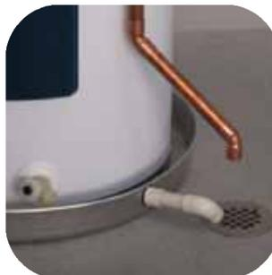
The Temperature and Pressure Relief Valve (T&P) discharge pipe should be terminated near a floor drain with an air gap of no more than 6 inches between the end of the discharge pipe and the drain. Some localities require terminating the T&P discharge pipe outside. In cold climates, we recommend using a floor drain. In all cases, follow the codes for your location. **Warning: Do not plug or cap the T&P discharge pipe.**
