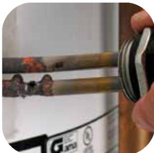
If you have no hot water (not even warm) after a few hours, check to make sure the water heater is getting power. If you have power but no hot water, the upper element may have been "dry fired" and will need to be replaced. Replacement elements are inexpensive and widely available.
