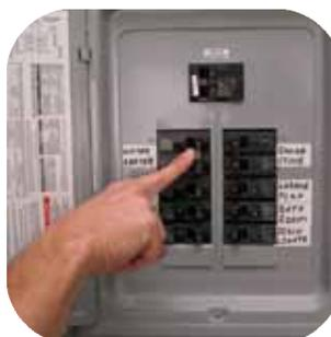
Turn the circuit breaker (or fuses) back on (and the disconnect if you have one). Because the tank is full of cold water, it may take several hours to reach normal operating temperature.
