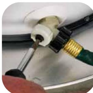
Connect a garden hose to the drain valve. Place the other end of the hose in a drain or outside (you could also use buckets). Open the water heater's drain valve. While the water heater is draining, read the Installation Instructions that came with your water heater. Disconnect the water and power lines and remove the old water heater.
