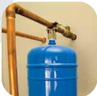
Almost all homes have check valves in the plumbing system and now need a thermal expansion tank installed near the water heater. The expansion tank is attached to the cold water inlet line. To operate properly, the expansion tank must be pressurized with air. Refer to the expansion tank's instructions for details.
