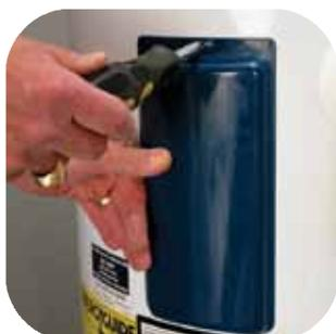
Replace the insulation, plastic protectors, and the upper and lower access panels. Replace the cover on the electrical junction box (on the top of the water heater).
