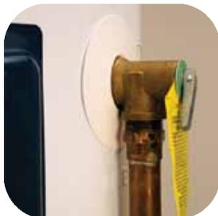
The Temperature and Pressure Relief Valve (T&P) is an important safety device. It opens to relieve pressure if the water temperature or pressure is too high. Use the new T&P that came with your new water heater. Don't reuse the old T&P valve.
