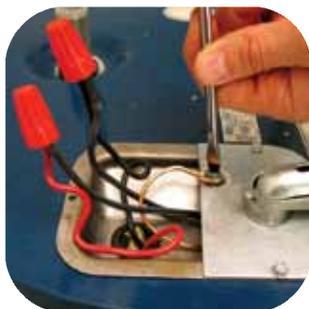
Consult the Installation Instructions and the wiring diagram and labels on the water heater. Make sure your home's wiring and circuit breakers are in good condition and are correct for the model you are installing. Connect the power wires and the green or copper ground wire. The ground wire must be connected to the water heater's green ground screw.
